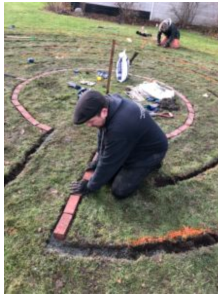
Laying the brick edging for the labyrinth. Image by Meagan Crosby-Shearer.
